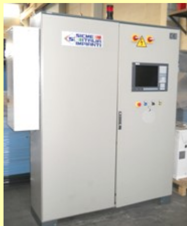
Main Electric control board
