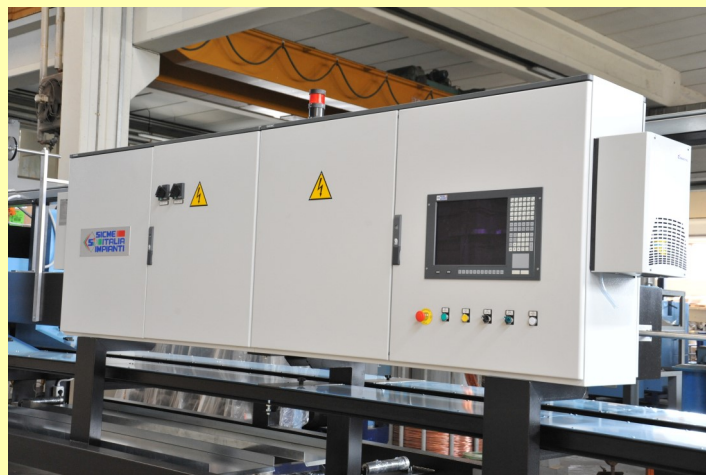
Main Electric control board
